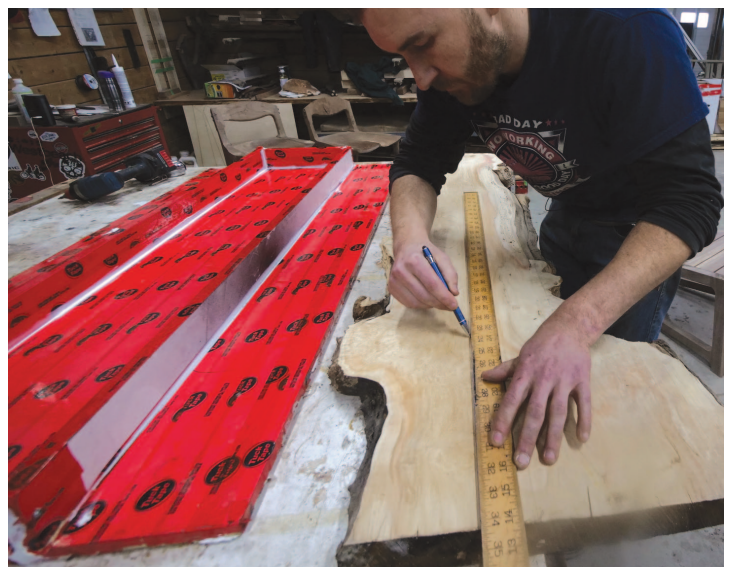
Mark the Lumber – Most lumber will need to be trimmed to size. Mark it with a straight edge, being sure the lumber will look good when matched with any other pieces you’re using, and will be sized appropriately.
